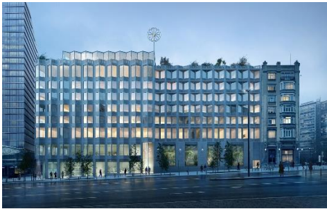
DoubleTree by Hilton Brussels City Operator Activities Extension of 151 rooms Completion expected in 2025 Investment: around MEUR 35
